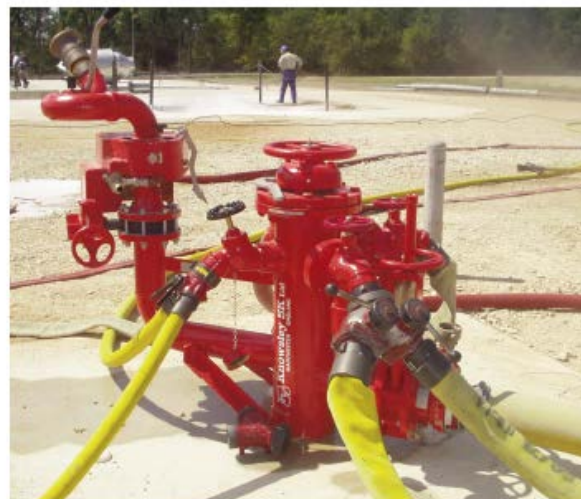
Figure 3 High Volume Pillar Hydrant with Oscillating Monitor
