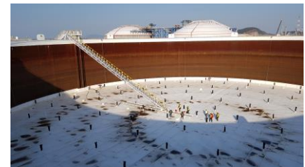
Floating roof of a storage tank
